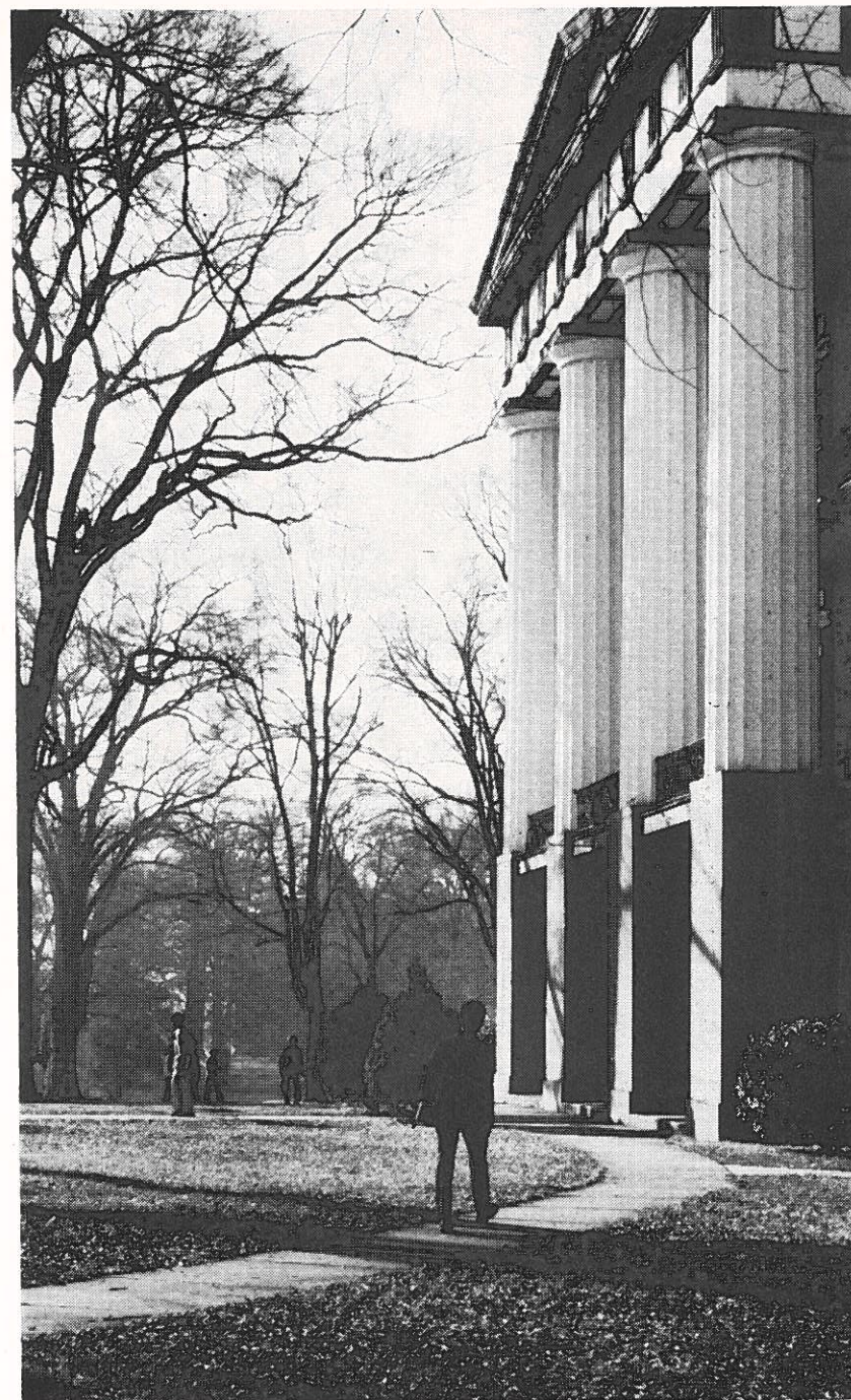
Historic Swayne Hall is the oldest building on campus.
